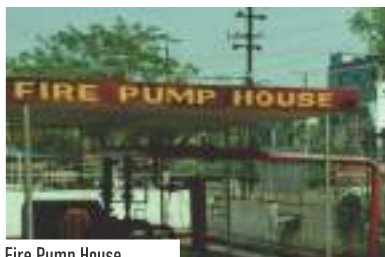
Fire Pump House
