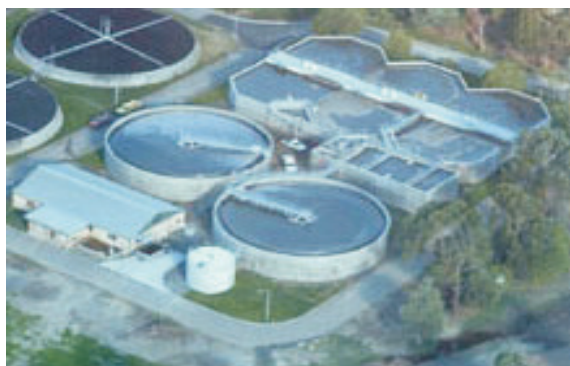
Figure 8.7 An aerial view of a sewage plant
