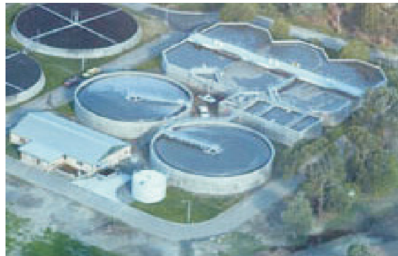
Figure 8.7 An aerial view of a sewage plant
