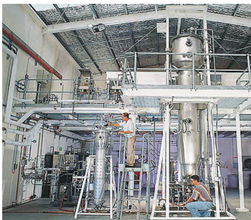
Fig. 8.5 (NCERT): A modern fermentation plant where industrial-scale brewing or antibiotic production happens. Stainless-steel pipework, jacketed vessels and aseptic transfer lines are the hallmark.
